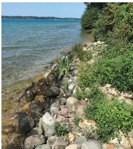
A successful revetment design that utilized stones of varying sizes, a slope that began beneath the water's surface, and incorporated appropriate plant material to increase resistance to wave energy.
